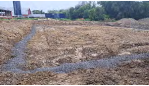
Dug Pit with perimeter trench
