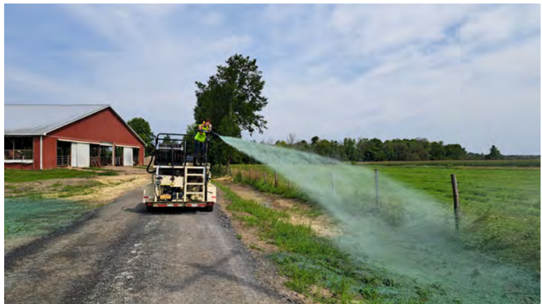
District staff hydroseeding the ditch near the new manure storage
